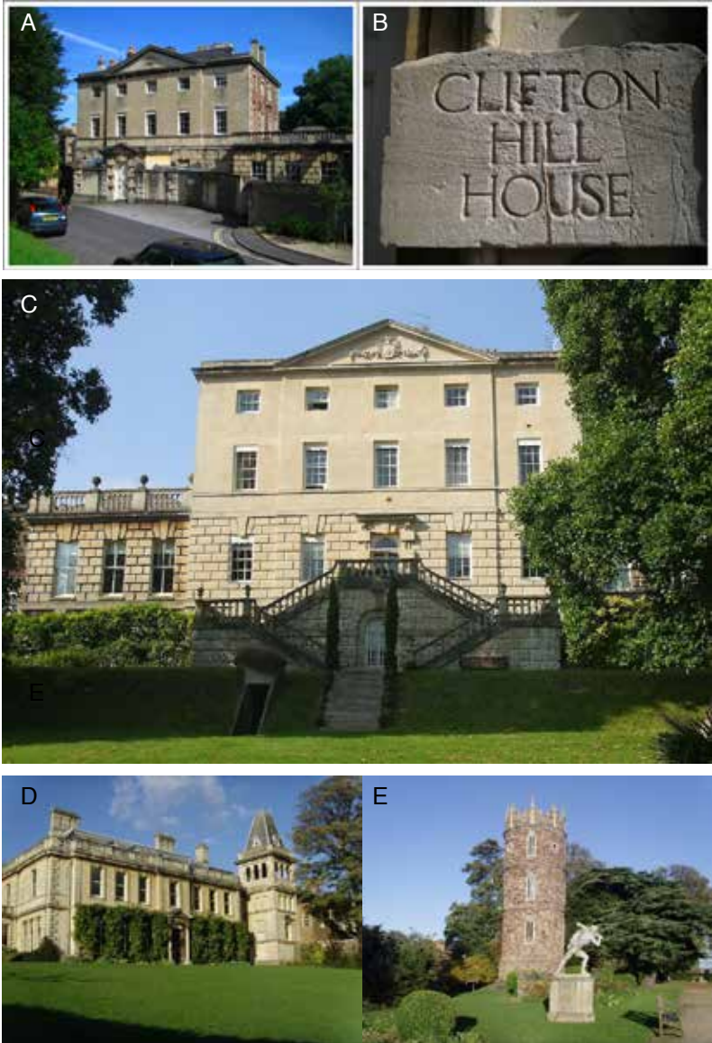
Figure 3. Two early Clifton mansions. (A–C) Clifton Hill House, showing the north face (A), a detail of the house name in cross-bedded Bath Stone (B), and the rear elevation (C). (D–E) Goldney House, showing the garden side in Bath Stone (D), and the tower in Brandon Hill Grit, with statue of Hercules (E). (Photos by Charly Stamper (A, B), Francium12 (C–E), the last three Wikimedia, CC BY-SA 4.0.)
