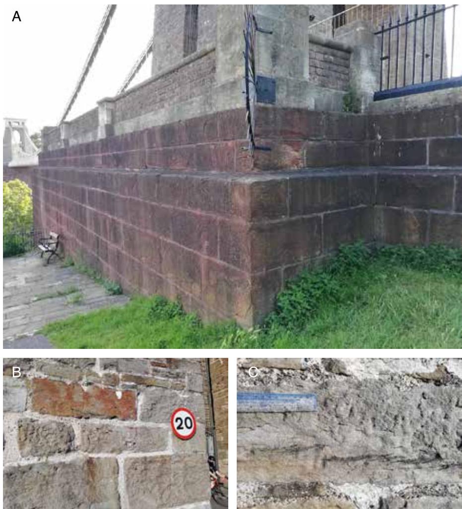
Figure 4. The building stones of the Clifton Suspension Bridge. (A) The abutments of the eastern end of the bridge. (B, C) Close-ups of Pennant Sandstone blocks in the tower, showing red mudstone clasts (B) and thin whisps of coal (C). ( Photographs by Michael Benton. )
