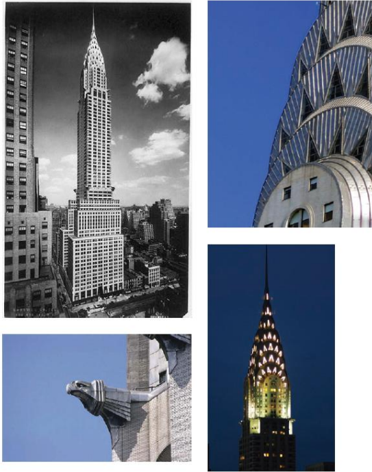
Chrysler Building , New York (1930), designed by William Van Alen Steel supported brick construction, stainless steel cladding on crown. Height: 318.9 metres, 77 floors.
